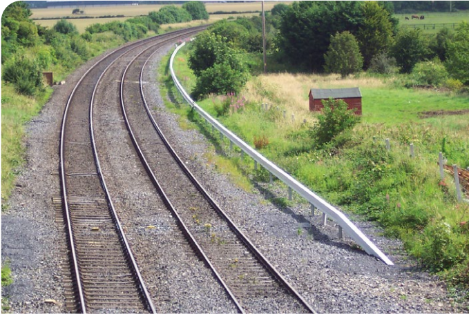
VARIO TOP size 2 along the track line
