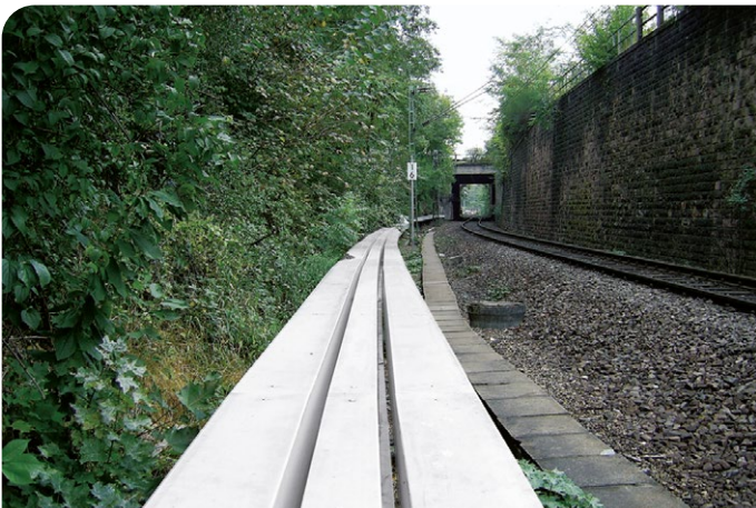
Three parallel cable ducts on one support
