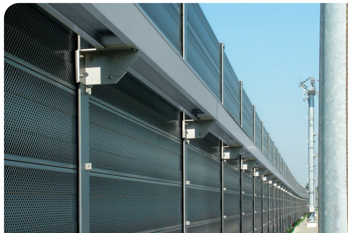
VARIO-TOP® size 2 – Special solution on a noise barrier
