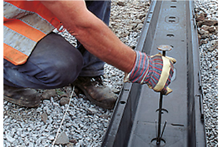
Fixation of the cable duct with specific ground anchors depending on local requirements
