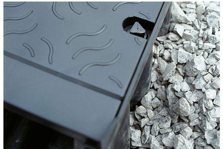
Filling of the cable ducts
